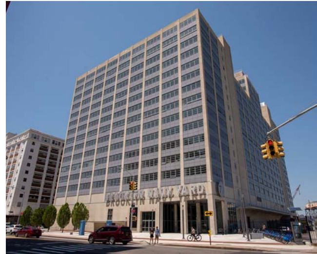
Building 77, Brooklyn Navy Yard.
